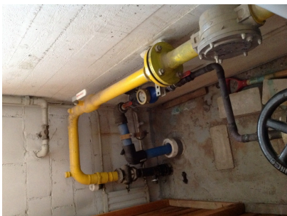
Main water cut-off valve in building 8
