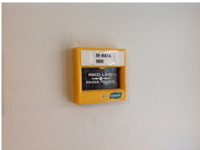
Air-conditioning emergency stop button
