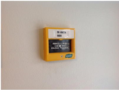
Air-conditioning emergency stop button
