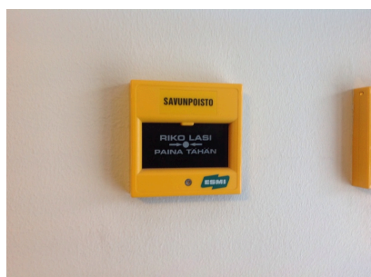
Smoke extraction activation button
