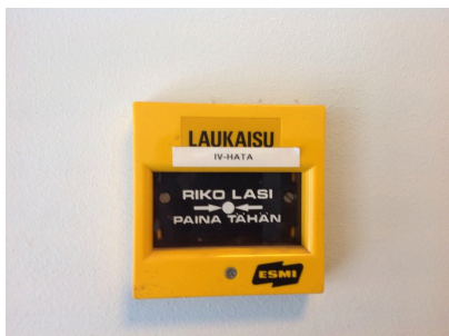
Air-conditioning emergency stop button
