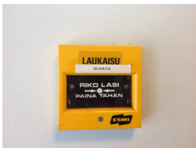
Air-conditioning emergency stop button
