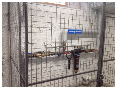
Water inlet shut-off
