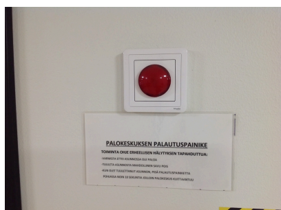
Acknowledgement button for the fire alarm centre
