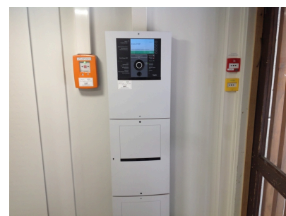
IV emergency stop, smoke alarm and smoke extraction triggering
