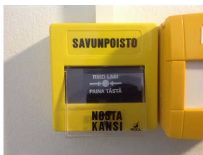
Smoke extraction activation button
