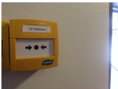
Air-conditioning emergency stop button
