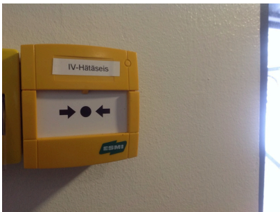
Air-conditioning emergency stop button
