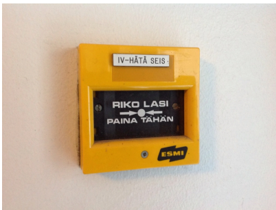
Air-conditioning emergency stop button
