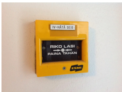
Air-conditioning emergency stop button
