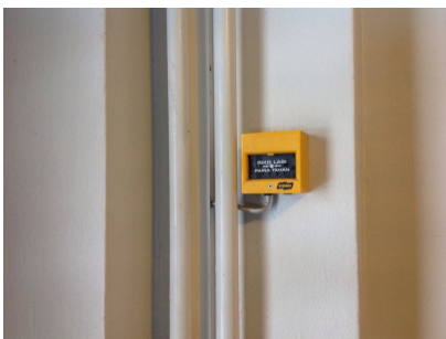
Air-conditioning emergency stop button
