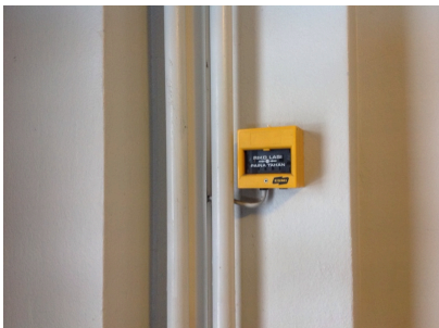
Air-conditioning emergency stop button
