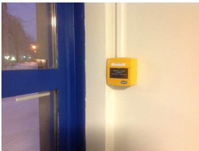
Air-conditioning emergency stop button
