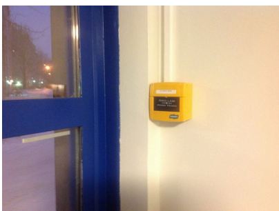
Air-conditioning emergency stop button
