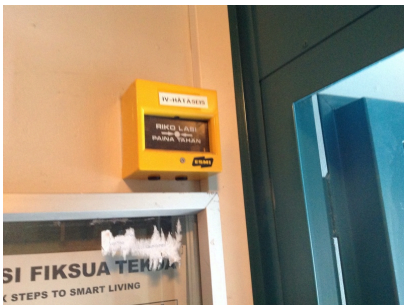
Air-conditioning emergency stop button
