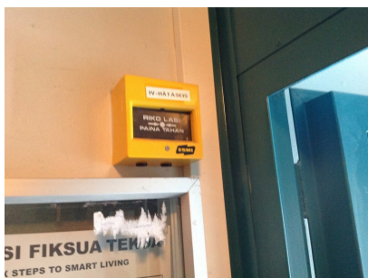
Air-conditioning emergency stop button
