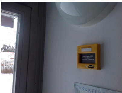
Air-conditioning emergency stop button
