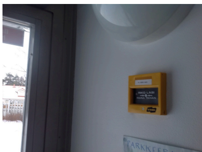
Air-conditioning emergency stop button
