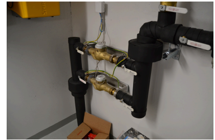
Main water cut-off valve
