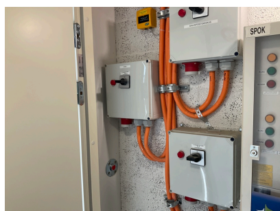
Second fire department stand-pipe lock, next to the smoke extraction centre
