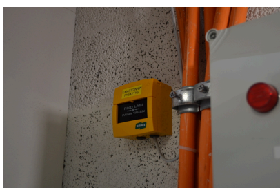
Air-conditioning emergency stop
