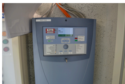
Fire alarm switchboard
