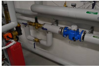
Main water cut-off valve
