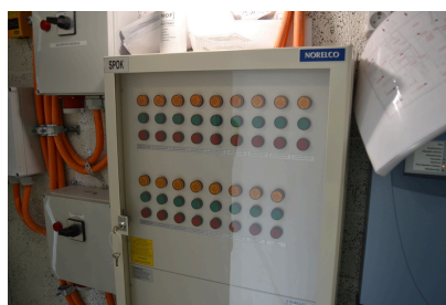
Smoke extraction activation panel
