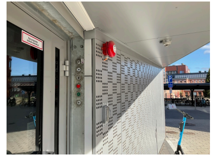
Standpipe locks and a fire siren by the front door
