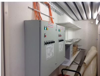
Smoke removal centres in the building storage room
