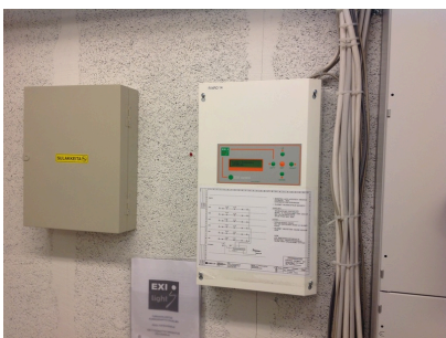
Emergency light centre in the electricity mains
