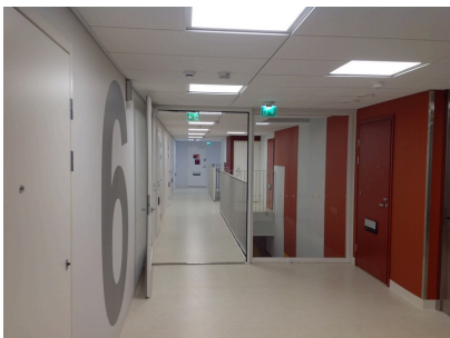
Fire barrier systems on the borders of the fire departments on each floor
