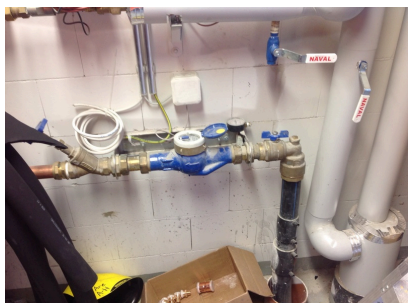
The water mains stop is located in the heat distribution room
