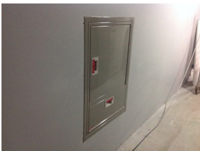
Quick fire hydrant with a first aid extinguisher cabinet
