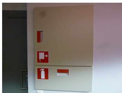
Initial fire extinguisher and fire hydrant
