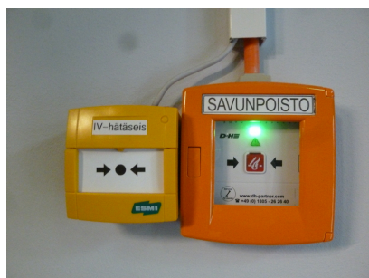
AC emergency shutoff and smoke extraction trigger
