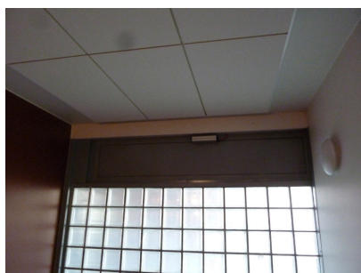
Smoke extraction hatch
