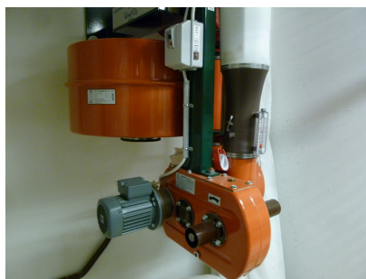
The air-conditioning apparatus of civil defence shelter 2
