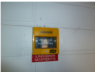
Air-conditioning emergency stop
