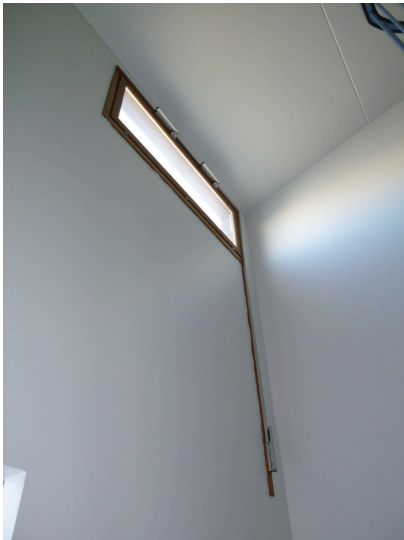
Smoke extraction hatch
