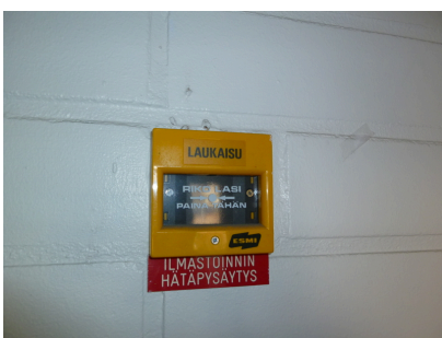
Air-conditioning emergency stop
